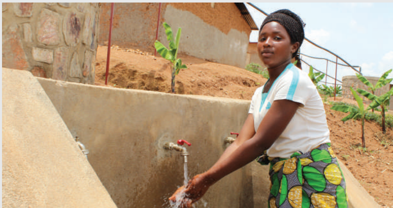
ActionAid Rwanda established six water harvesting tanks
